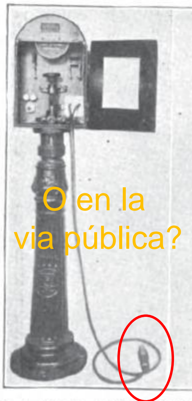
FIGS. 1 AND 2—CURB CHARGING STATION FOR ELECTRIC AUTOMOBILES
