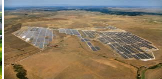
Trujillo, Extremadura, Spain-Elecnor 23 MW SunPower T0 Tracker
