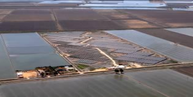
Isla Mayor Spain, 8.4 MW SunPower T0 Tracker
